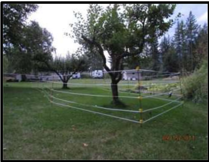
Figure 17. A five-strand portable electric fence set up to deter grizzly bears. Photo courtesy of Gillian Sanders.
