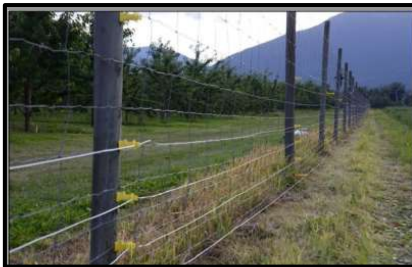
Figure 19. Ensure that vegetation below electric fence is removed or kept below wires. This is a 5-strand electric fence modified to fit with an existing page-wire fence. Photo courtesy of Gillian Sanders.
